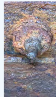
Steep Creek Bridge - Uncoated
