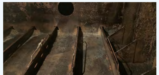
Ballast tank coated in S2S
